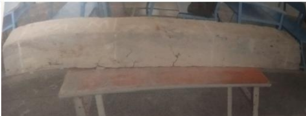
Figure 9. Failure pattern of S4 Specimen
