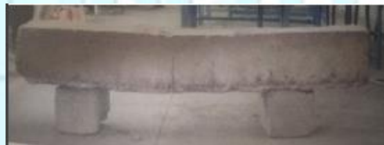
Figure 4. Failure pattern of S1 specimen
