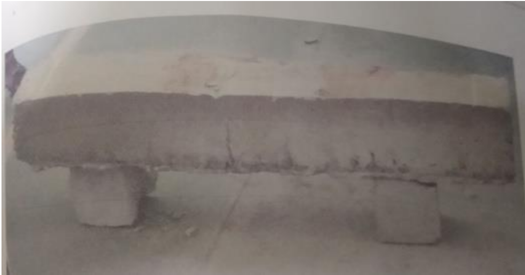
Figure 12. Failure pattern of S5 specimen
